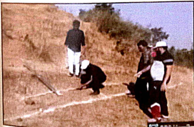
Drawing the lines of ground for Continuous Contour Trench (C. C. T.) Technique
